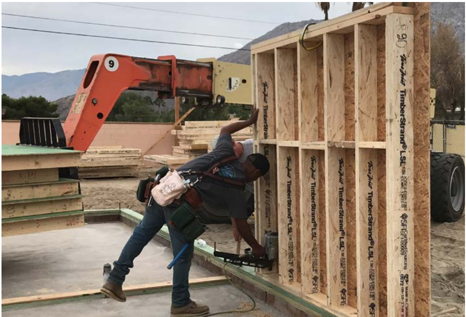
Laminated Strand Lumber and Oriented Strand Board
