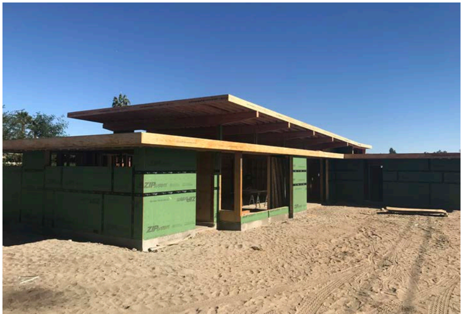
Assembled Structure of Prefab Package
