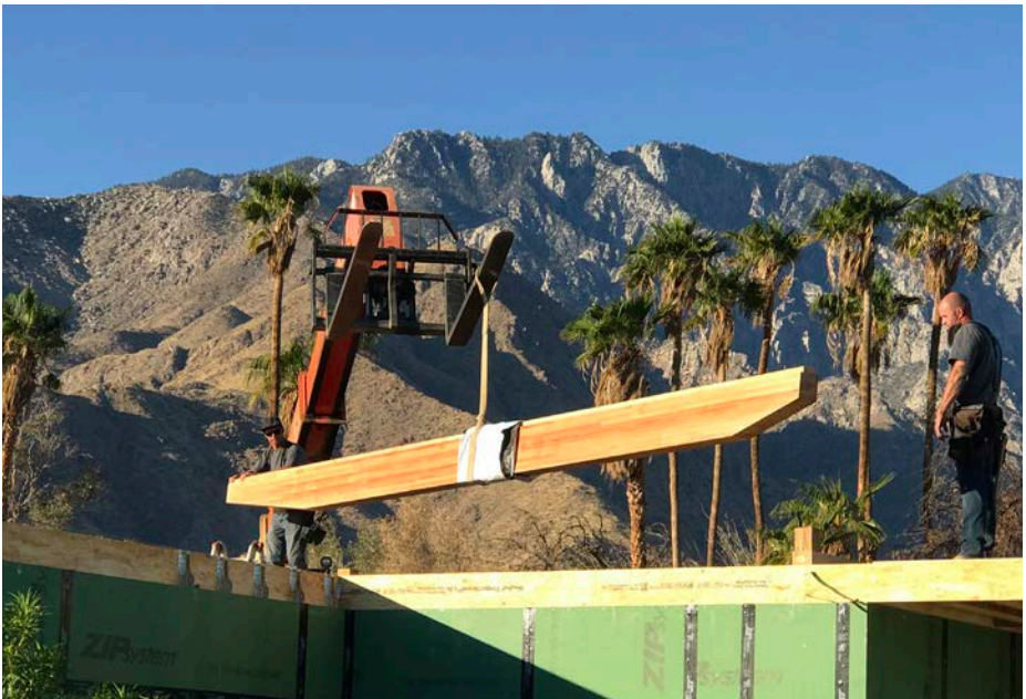
Laminated Douglas Fir Beams, with Structural Old Growth Veneer
