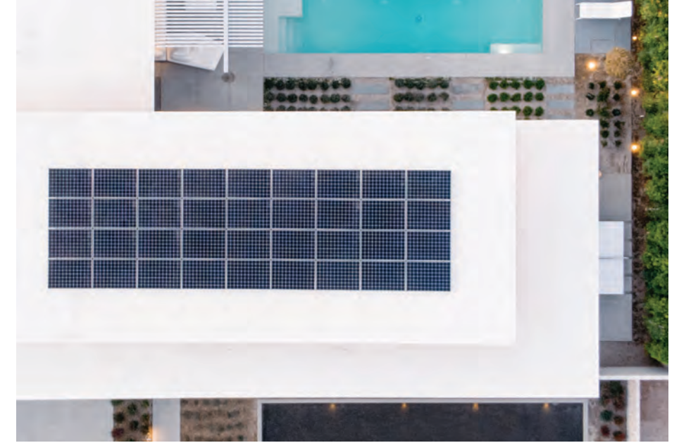
36 Installed Solar Panels
