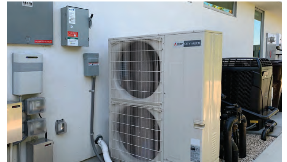
Heat Pumps, On-Demand Hot Water Heater, Etc.
