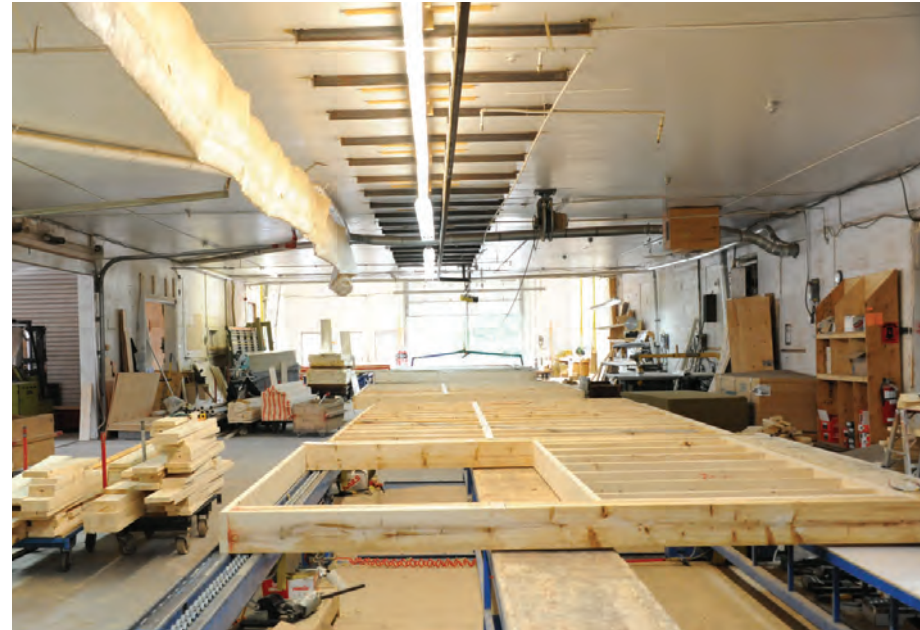
Wall Panels Built in a Factory
